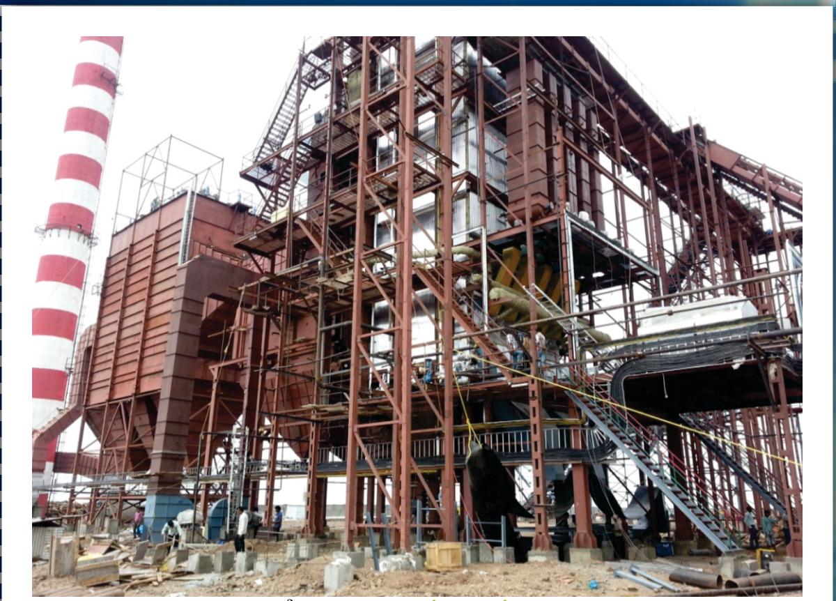
70TPH At 78 Kg/cm 2 Temp - 510°C ± 5°C (M/s. Sadguru Sugar)
